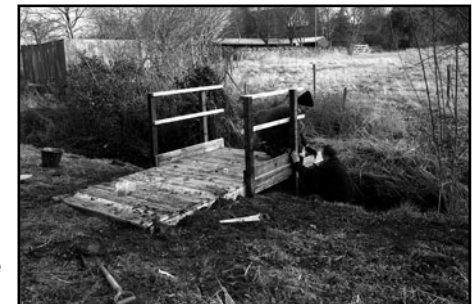
Installation of the pond dipping platform
