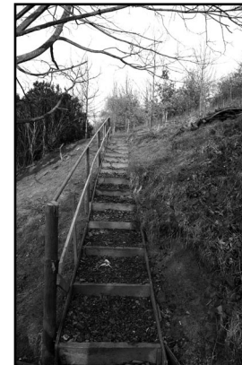
Installation of the new foot path
