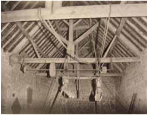
Hay barn roof trusses
