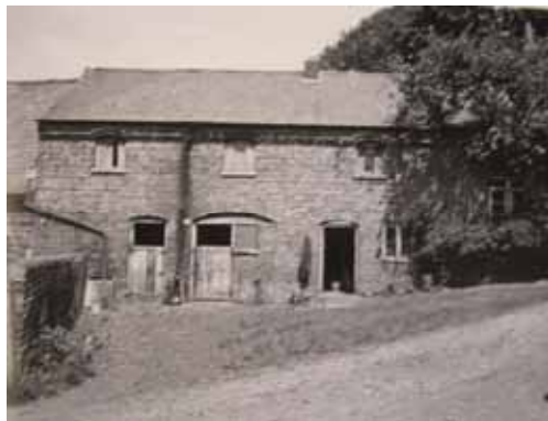
New stables & Mrs Burman's cottage now entrance lobby to High barn
